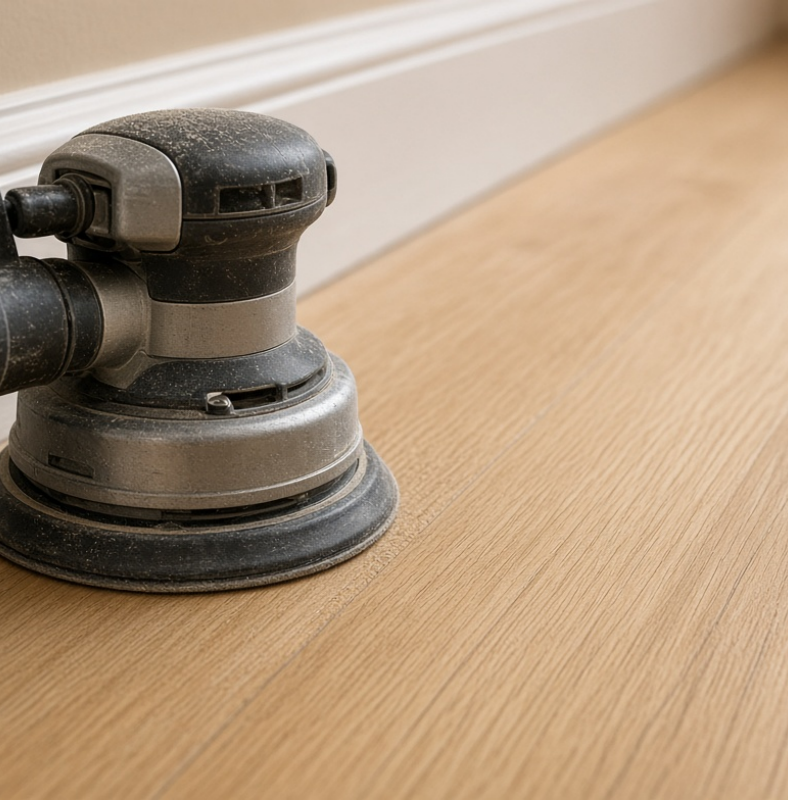
Perimeter work · edger, then hand-blend
